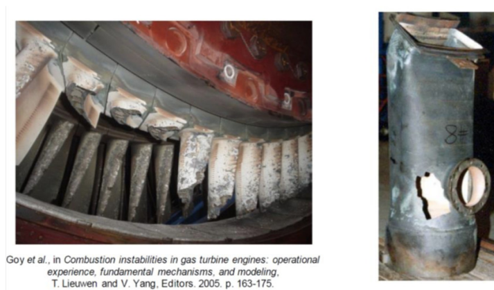
Figure 1.4: Structural damage of turbine first stage stator, and liner transition piece for a stationary gas turbine engine due to thermoacoustic combustion instabilities. Reproduced from [1].
